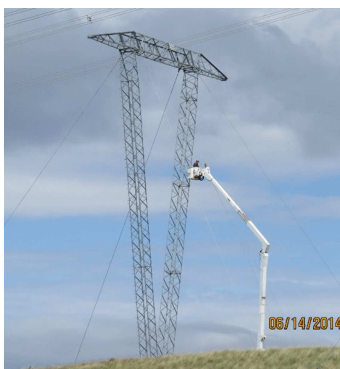
Lattice Guyed Flat Tangent (most PGGT towers)
