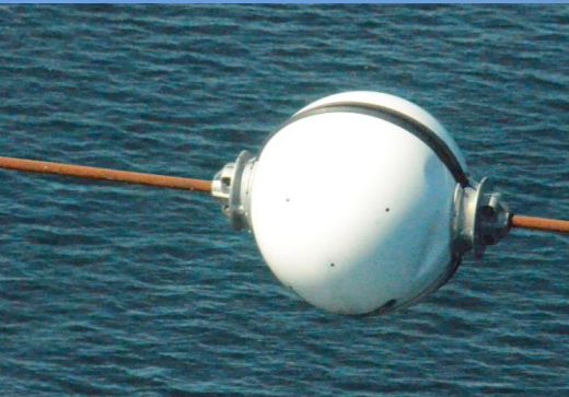
Aviation marker ball replacement.
