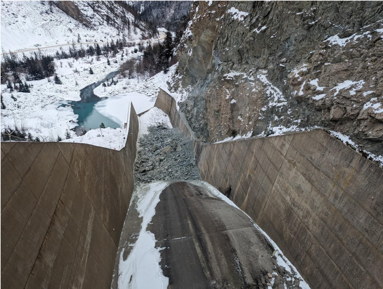
Figure 2 – Rockfall in the lower spillway chute at Terzaghi Dam (January, 2024).
