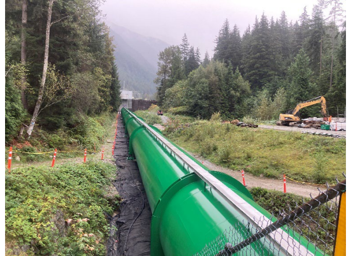
Figure 12 Recoated penstock at Lake Buntzen 1 Generating Station.
