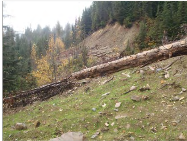
Photo 11. Deactivated section of the Westfall FSR, October 15 th , 2014.
