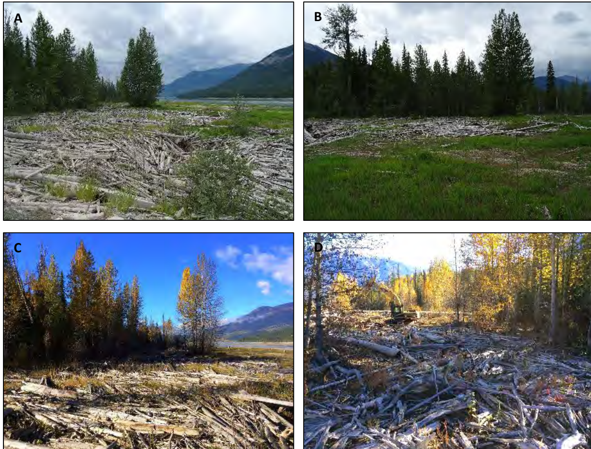
Figure 4-1: Examples of vegetation cover and wood debris distribution at the Bush Arm Causeway South site prior to construction in summer 2015 (A and B) and during construction in the fall (C and D). Summer photos dated July 15, 2015; fall photos dated Sept. 28, 2015.
