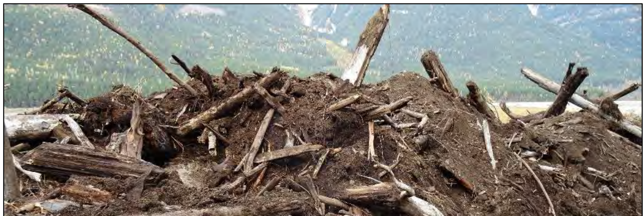
Figure 4-5: The completed mounds at the Bush Arm Causeway south location showing the matrix of substrate and woody debris with a rough surface.
