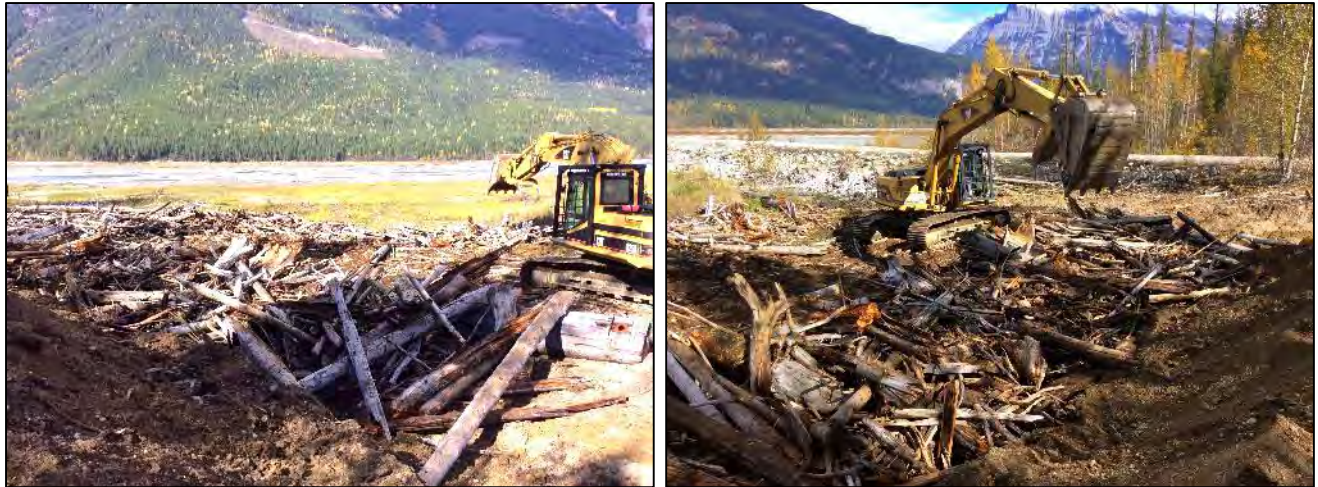
Figure 4-4: Filling the 'nest' with smaller logs, debris and soil.
