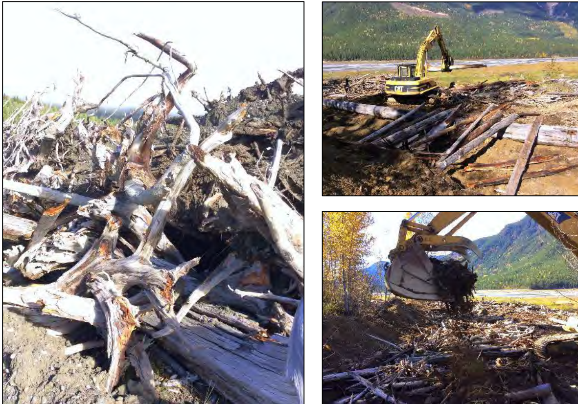
Figure 3-1: Examples of root wads used in mound construction (left), placement of sill log (to anchor the mound) and cross pieces (top right) and filling in excavation with small woody debris and soil (bottom Right).
