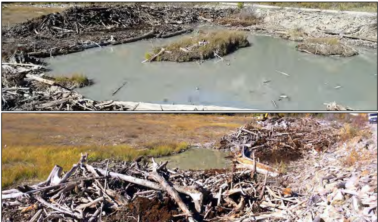
Figure 4-14: Some of the completed mounds at the Bush Arm Causeway north location showing the height of the mounds relative to the existing causeway. In this locations mounds were built perpendicular and parallel to the existing roadbed.
