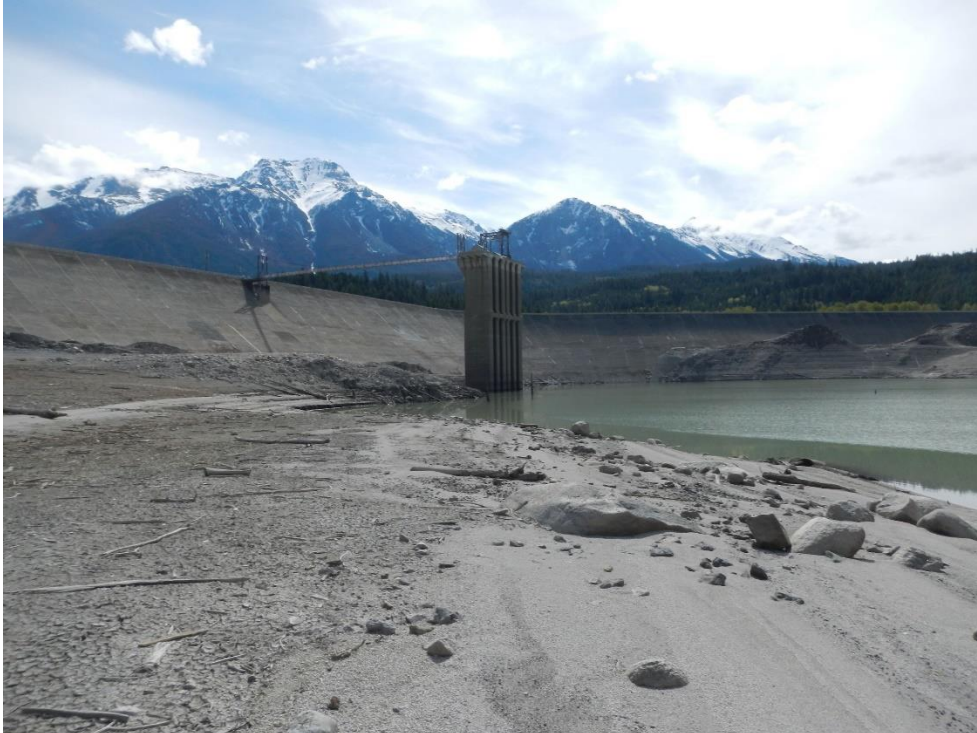
Photo A7 Reservoir Habitat Type 5: Dam Face (at approx. 722 m elevation). Note the reduced reservoir-dam interface (and exposure of natural substrate materials at the toe of the dam) at lower elevations relative to Photo A6.
