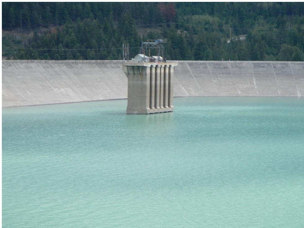
Photo A6 Reservoir Habitat Type 5: Dam Face (at approx. 734 m elevation)
