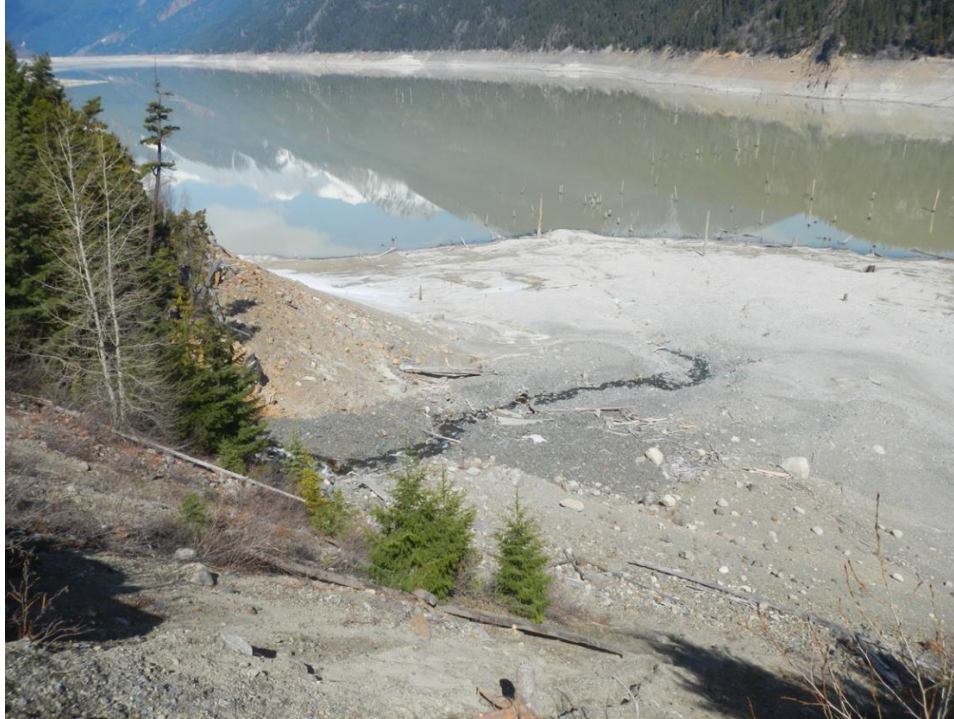
Photo A10 Ault Creek observed flowing to ground at a reservoir elevation of 712.5 m on 19 April, 2018.
