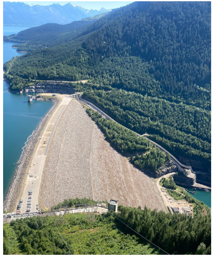
Mica Dam and Kinbasket Reservoir
